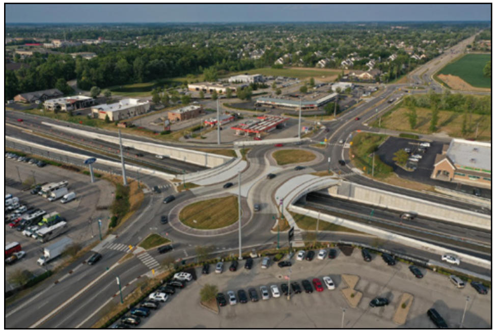
Photo courtesy of American Structurepoint
