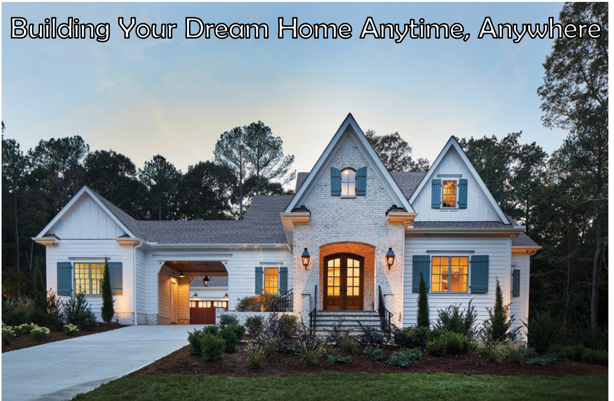
Photo courtesy of Laury Glenn and Paragon Building Group
