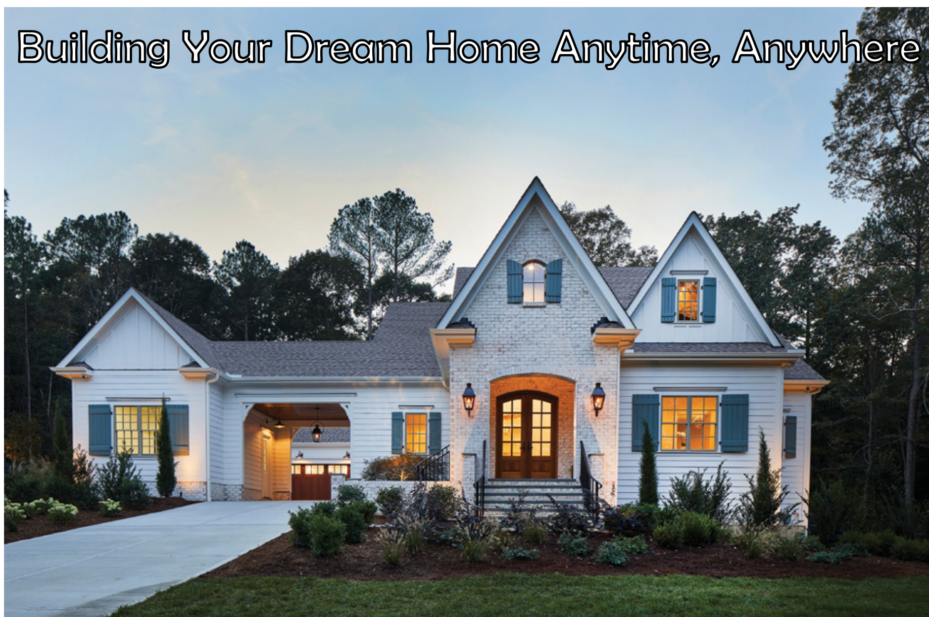
Photo courtesy of Laurey Glenn and Paragon Building Group
