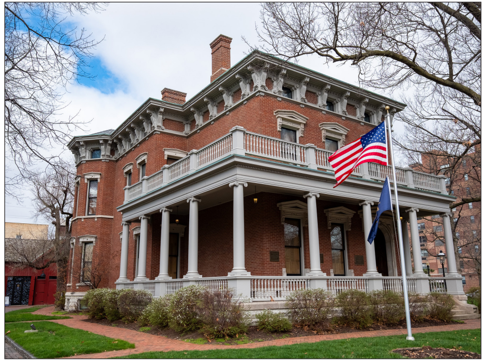
The Benjamin Harrison House, Indianapolis
